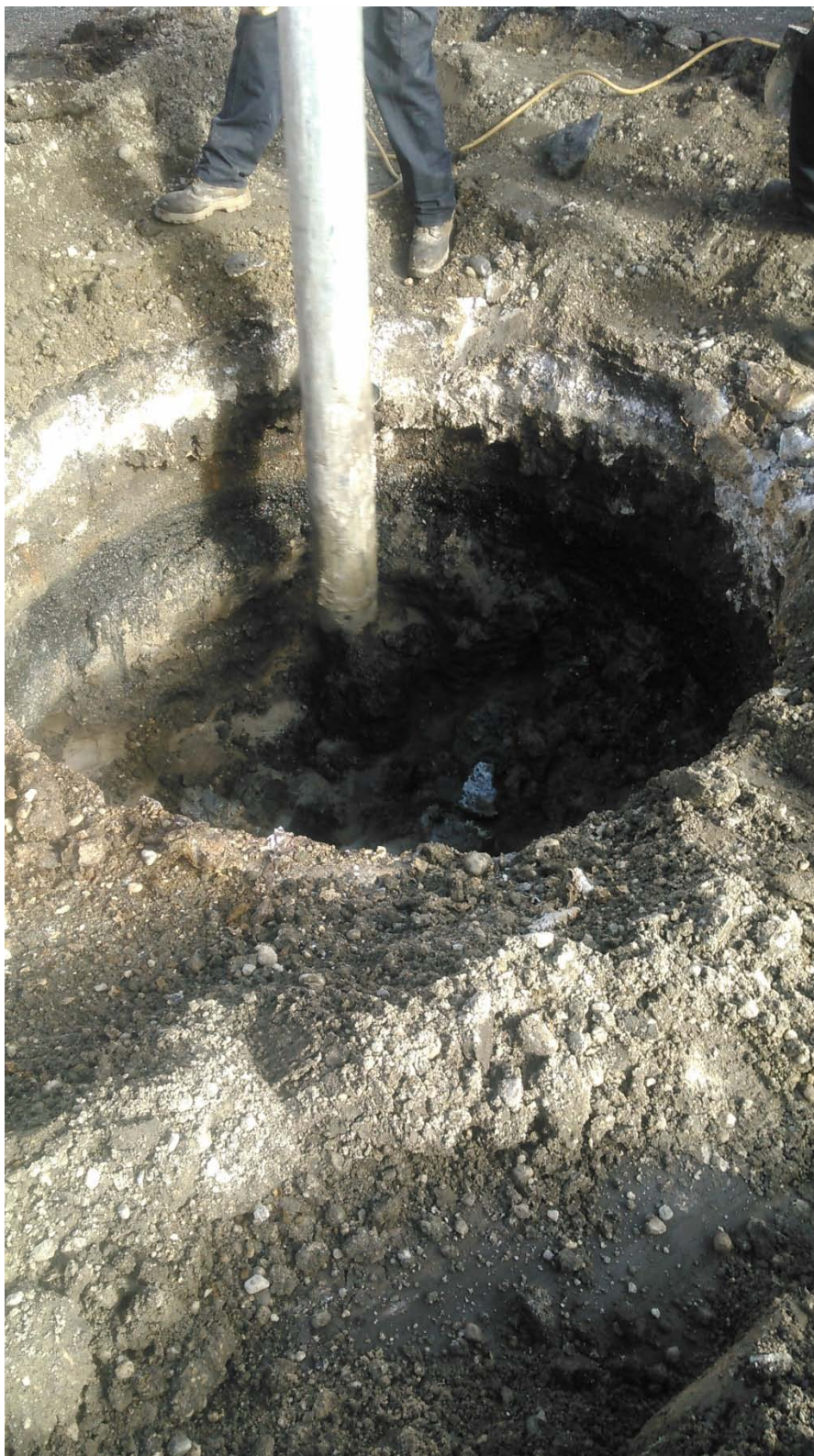
UIC Remediation at 300 Long Island Avenue Wyandanch, NY
