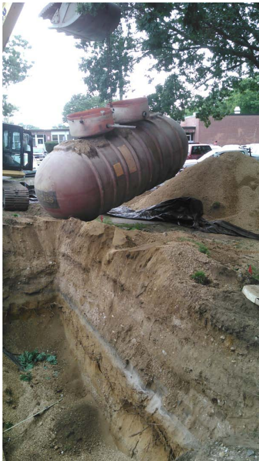
Tank removal by the Town of Babylon at a Town facility
