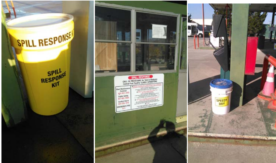
BMPs Implemented at the Town of Babylon Central Fuel facility Spill Response Kit, Signage and Speedy Dry
