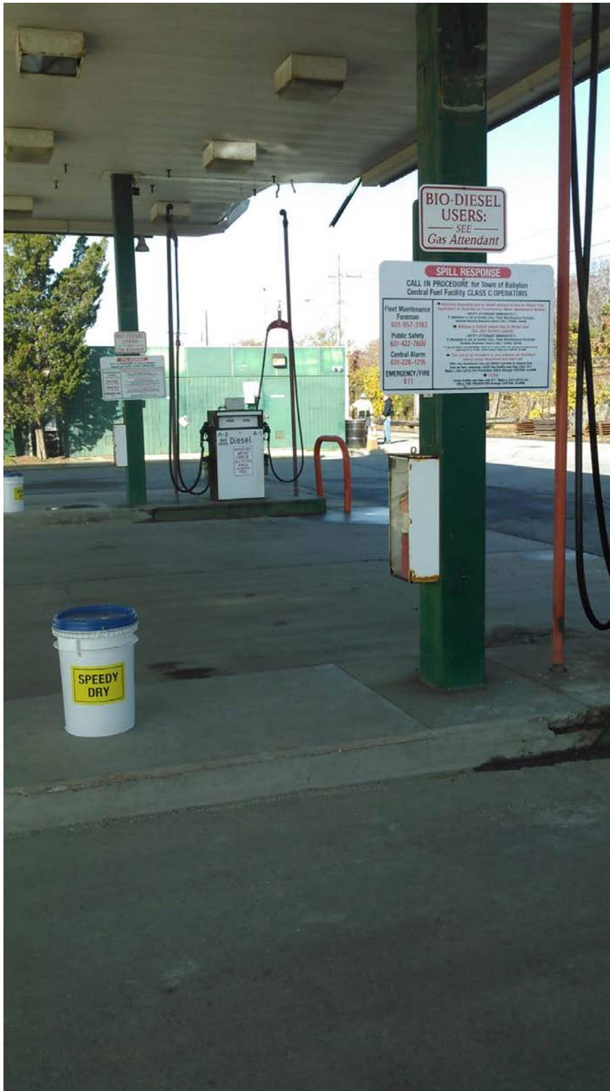
BMPs Implemented at the Central Fuel facility Speedy Dry and Signage
